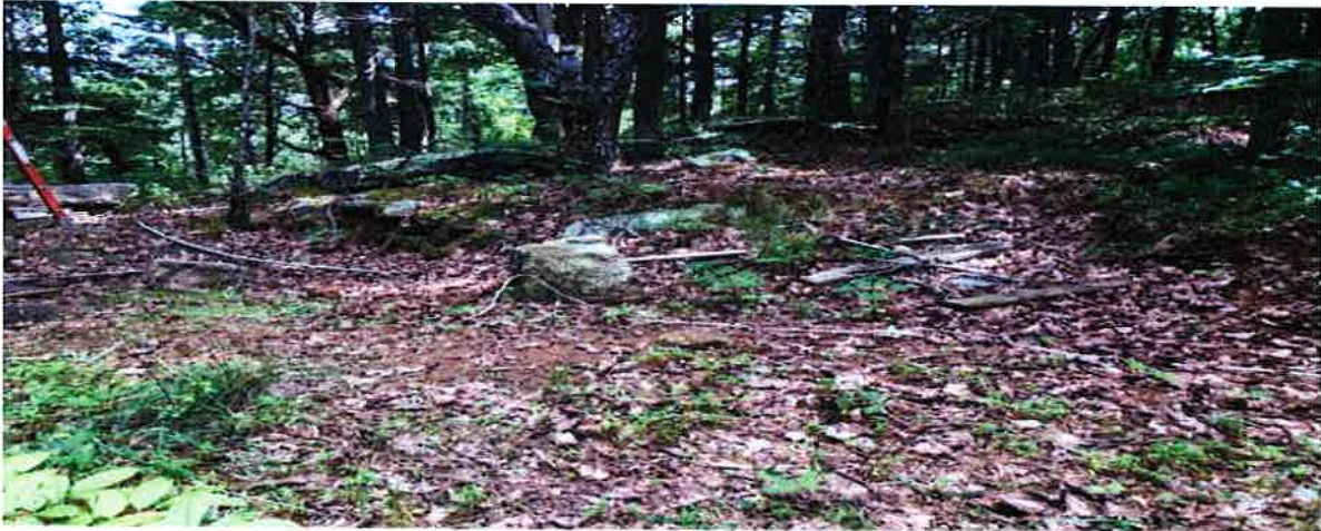
Bare wires on the ground that have no protection around them.
