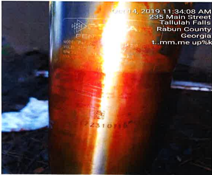
The Current Motor is in good shape which is a 5/8hp motor manufactured by Pentair
