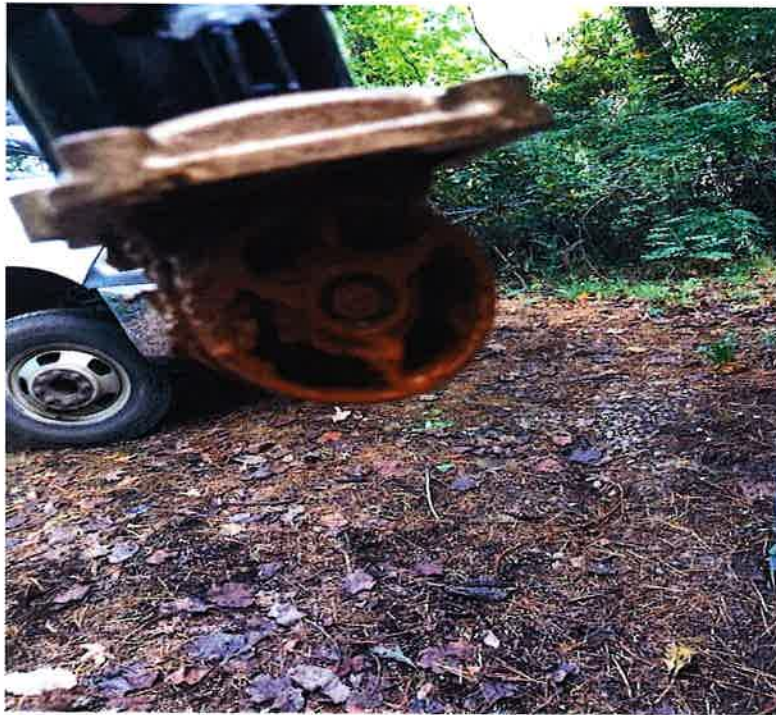
This picture shows the exit side of the flow meter again with the iron sludge.
