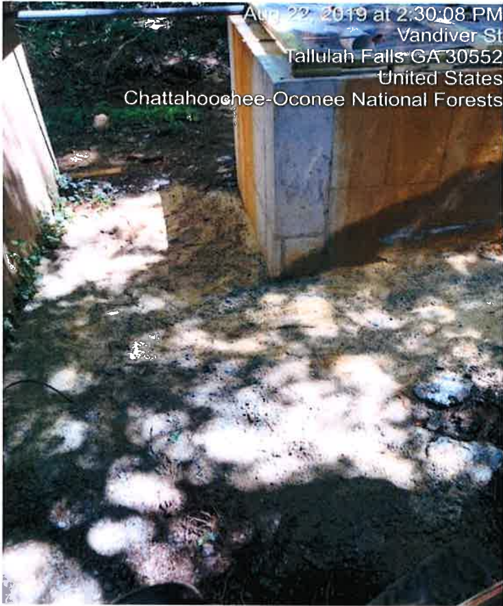
Picture 8. Soils have been cleaned around the outside structure.
