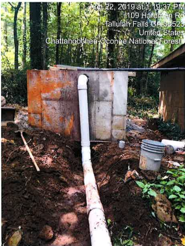
Picture 1. Hole has been cored and discharge pipe installed.
